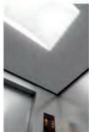
Ceiling: Painted steel sheet with a milky white resin lighting cover Lighting: Central lighting
